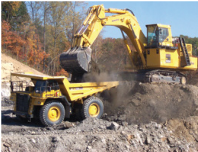
Kokosing’s heavy equipment on a mass excavation project.
