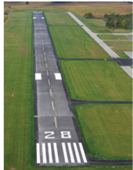
Kokosing Asphalt Division paved Knox County Regional Airport Runway.
